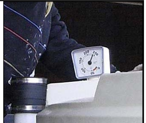
Fig 3.29 - Level Gauge, Fernery Tank
