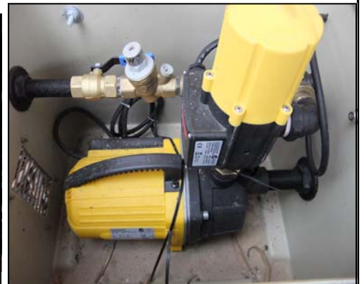
Fig 3.30 - Pump set with cover removed
