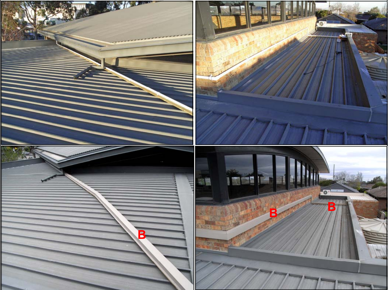
Fig 3.23 - White PVC Piping with covers
