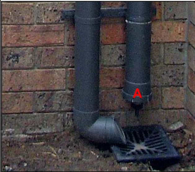
Fig 3.20 - First Flush Diverter (A)
