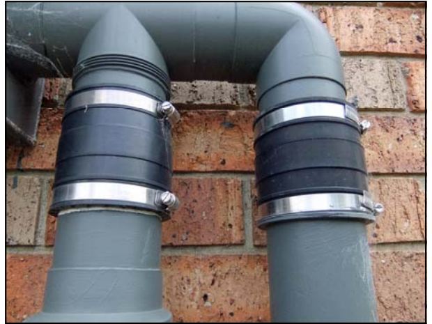
Fig 3.24 - Rubber Couplings with pipe clamps
