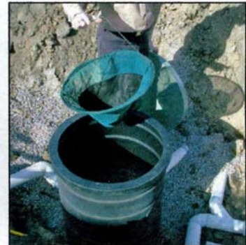
The trash screen collects all gross pollutants and micro pollutants as small as 180 microns.
