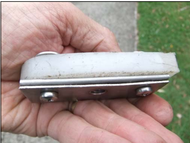
Fig 3.14 - Captive Nut for Pit Lid locking
