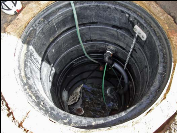
Fig 3.15 - View into installed pit
