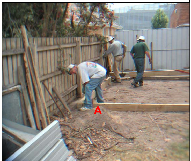
Fig 1.26 - Preparation of Tank foundation
