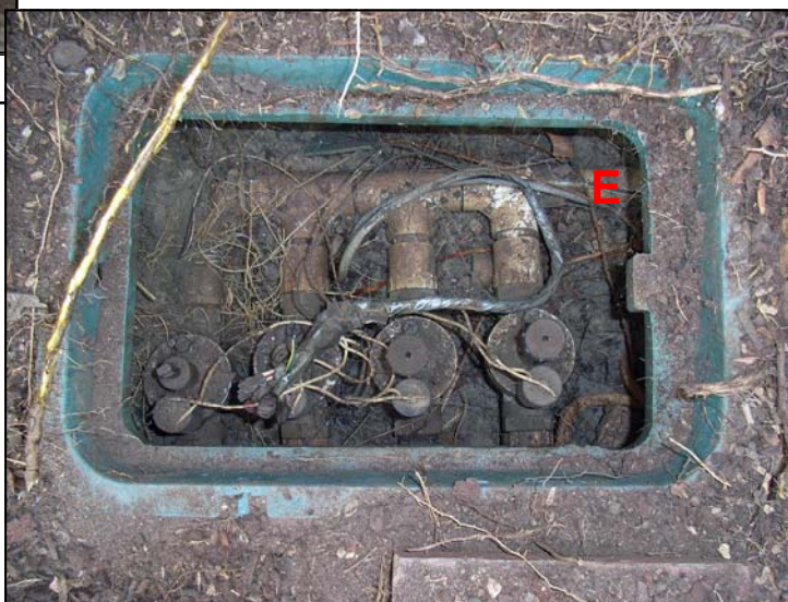
Fig 1.66 - Garden Watering East , 4 Solenoid Valve Pit
