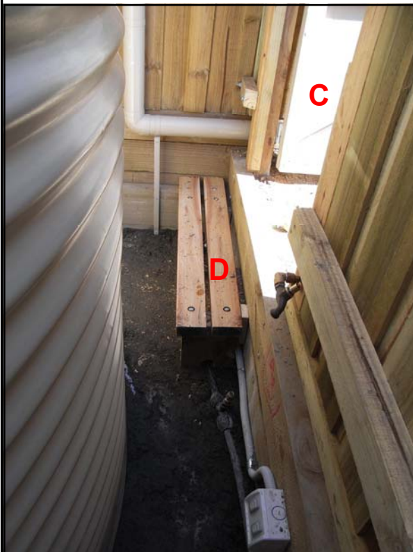
Fig 1.42 - Part of Manse enclosure
