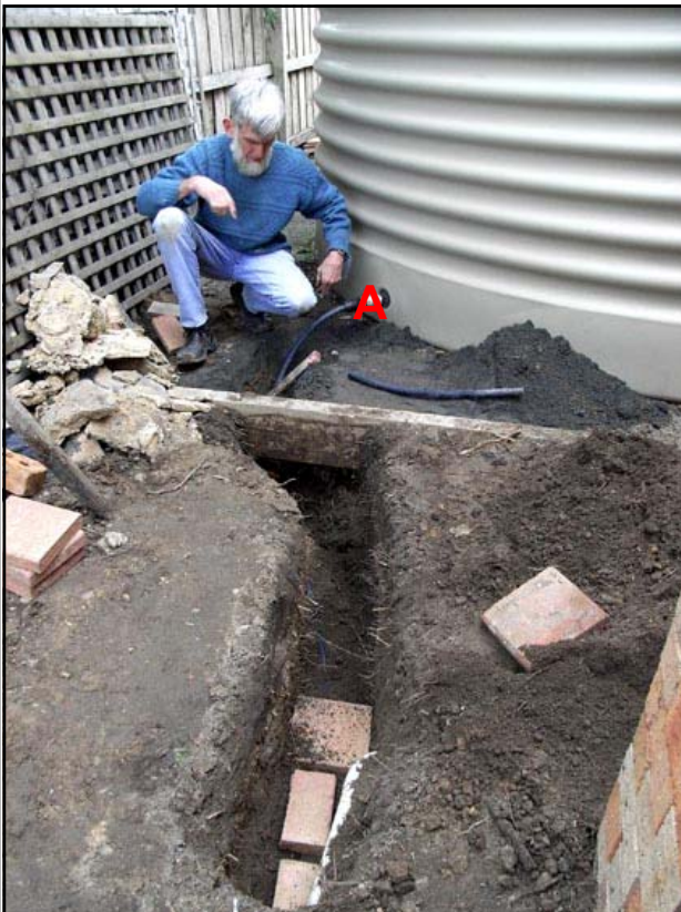
Fig 1.33 - Gravity Line from West Tank
