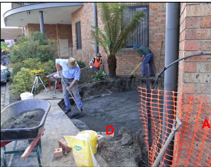
Fig 1.53 - Excavation & compacting, Fernery Tank
