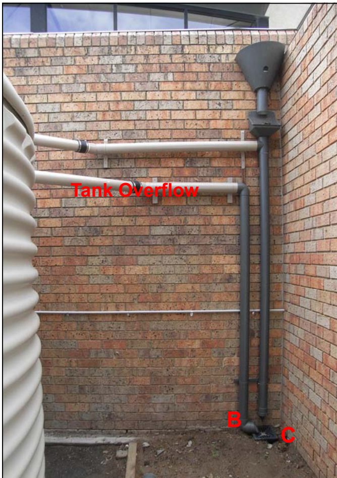
Fig 1.28 - West Tank overflow & stormwater drain
