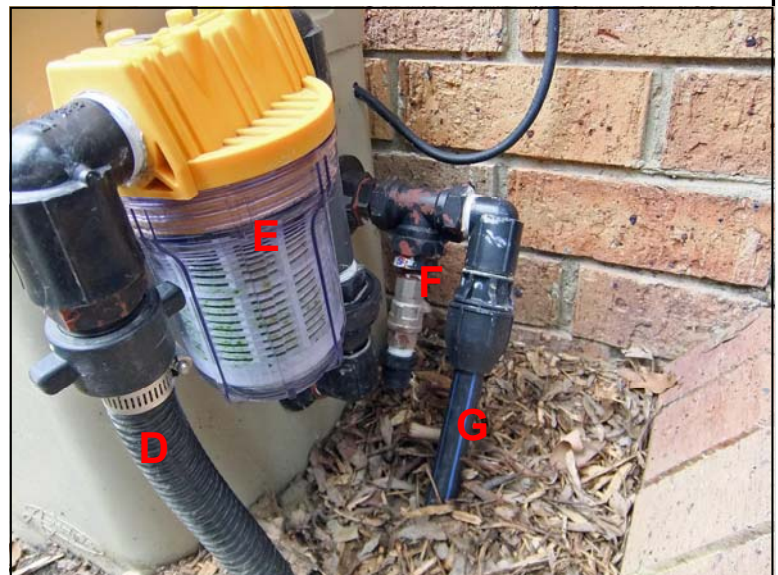
Fig 1.60 - Fernery Pump with cover removed
