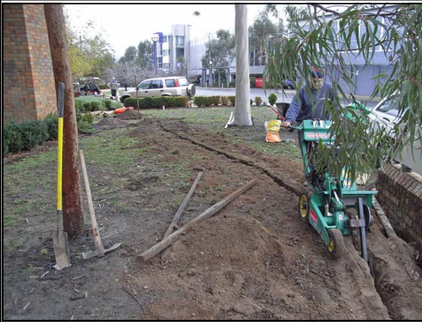
Fig 1.4 - Trenching across the Bogong Avenue side Lawn
