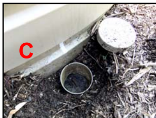
Fig 1.57 - Tank outlet
