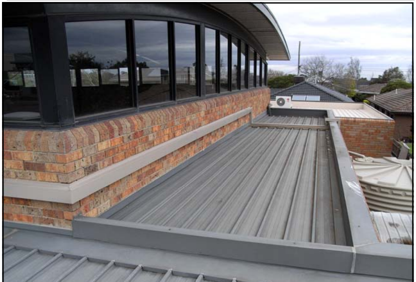
Fig 1.8 - Pipe route around Hall west wall
