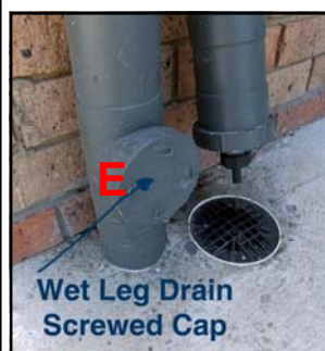
Fig 1.37 - Wet Leg drain
