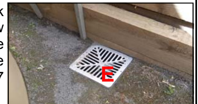
Fig 1.39 - Storm Water Pit, Manse Tank area
