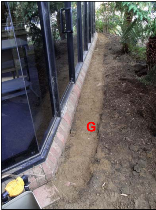
Fig 1.61 - Pipe route from Pump
