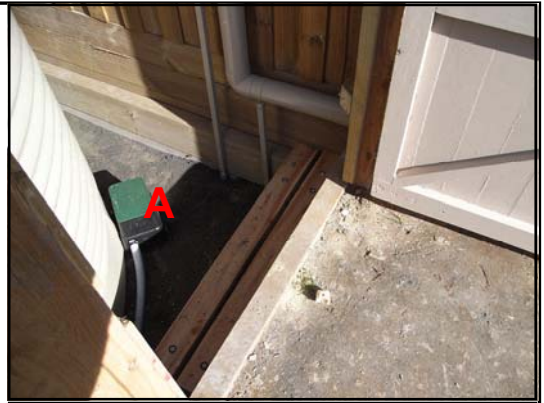
Fig 1.43 - Entry into the Manse Tank enclosure, and Tank Outlet
