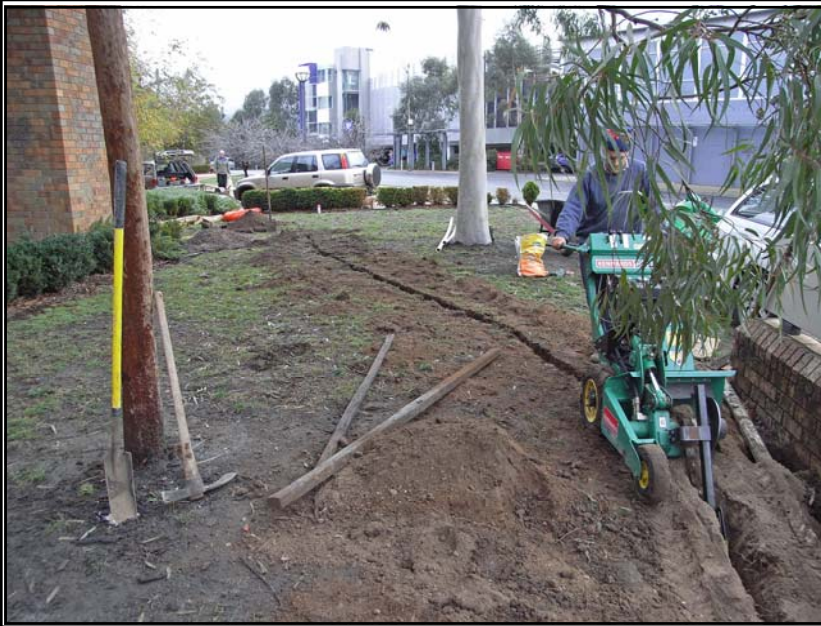
Fig 1.4 - Trenching across the Bogong Avenue side Lawn
