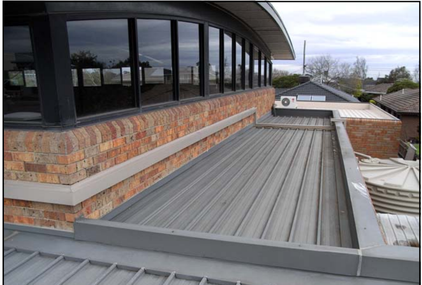
Fig 1.8 - Pipe route around Hall west wall
