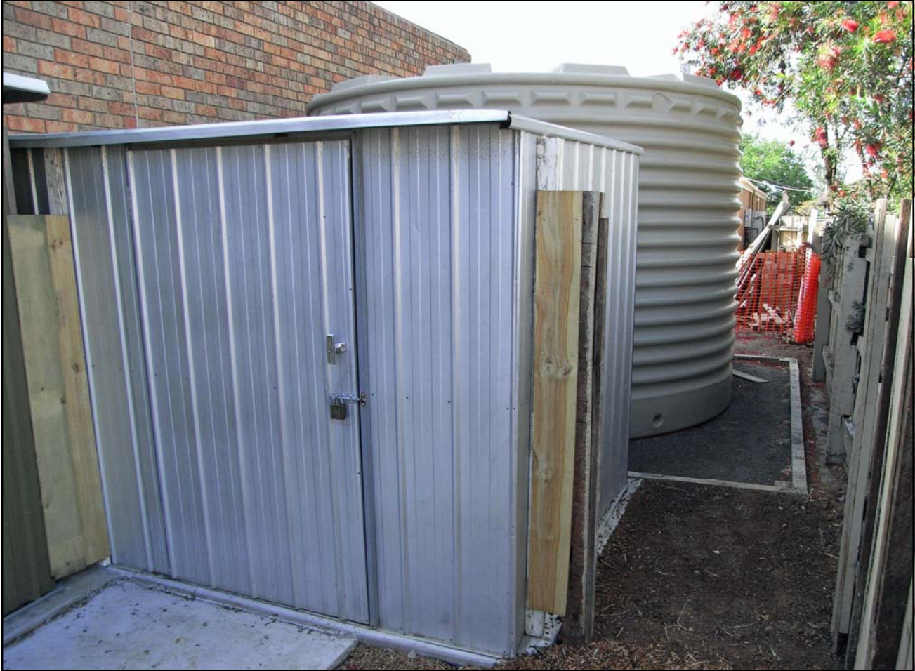
Fig 1.25 - West Tank, 22,000 Litres
