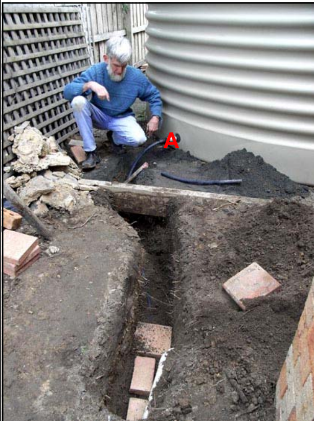
Fig 1.33 - Gravity Line from West Tank
