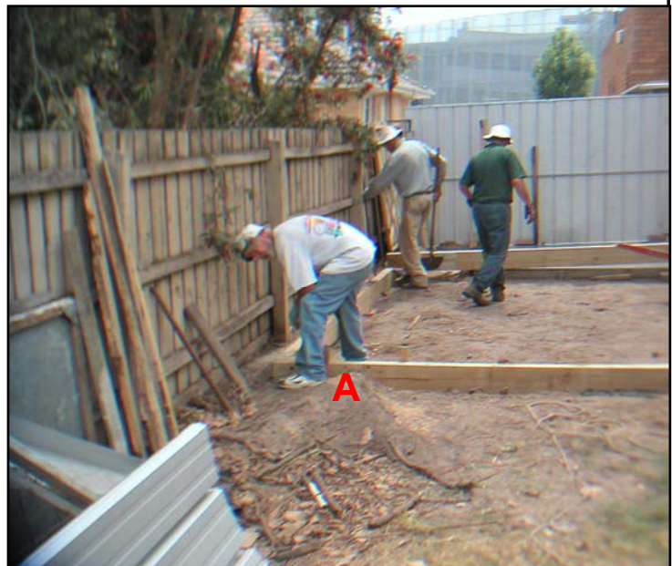
Fig 1.26 - Preparation of Tank foundation
