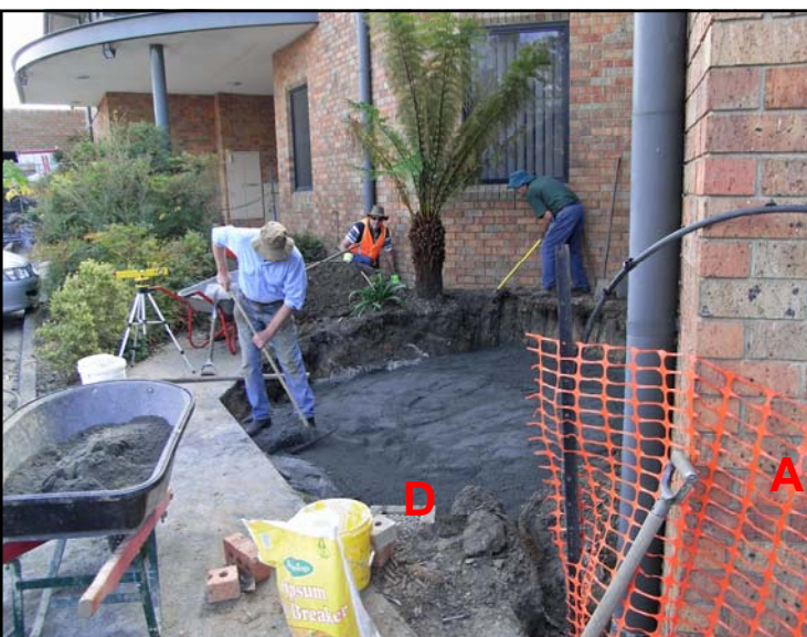
Fig 1.53 - Excavation & compacting, Fernery Tank
