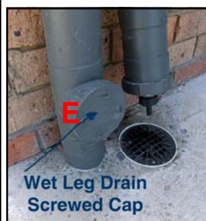
Fig 1.37 - Wet Leg drain
