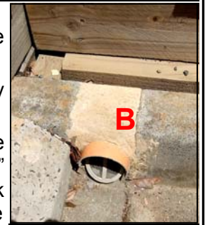
Fig 1.41 - Manse Tank Overflow
