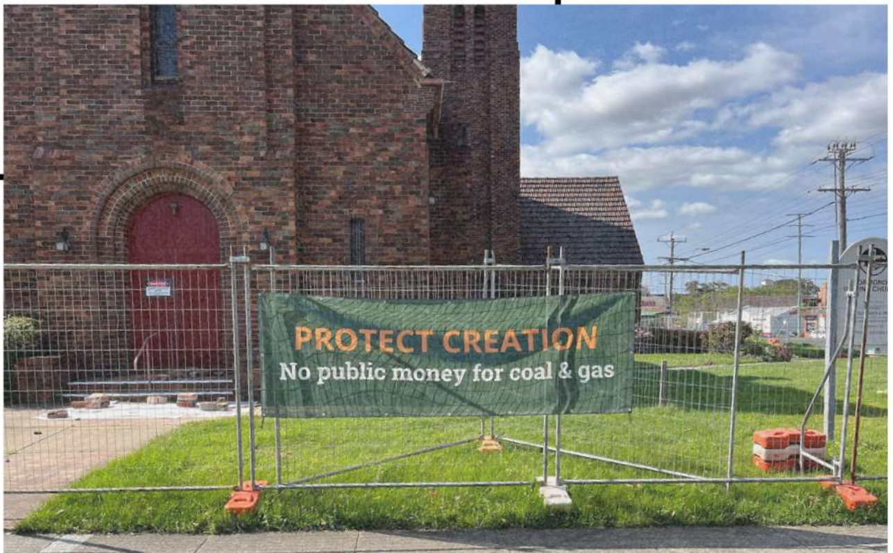
Banners by the Australian Religious Response to Climate Change, displayed at Ormond Uniting Church as it undergoes renovations.
